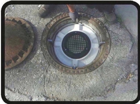
Image3 - The sponge seal closes the gap between the filter and manhole.
