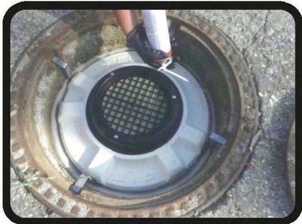
Image 4 - Small gaps around the filter are filled with polyurethane foam.
