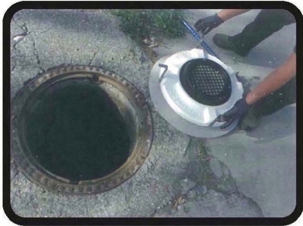
Image 2 - Easily placed under the manhole cover with hooks.
